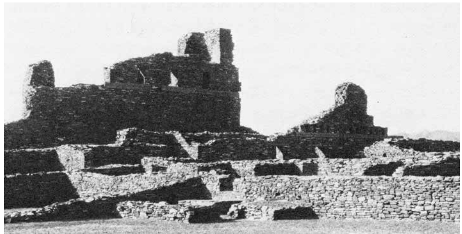
The Abó Mission, built in 1646, had extensive friary and support buildings, a fine organ and choir, and supervised the lives of 300 Indian families. The Indians were also used as beasts of burden by the civil authorities for the transport of salt.
