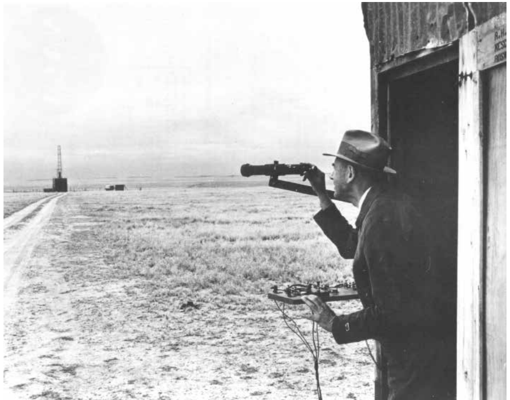
Robert Goddard reads pressure and lift gauges at the tower through a telescope. At his fingertips are three telegraph keys used to trigger launch events.
